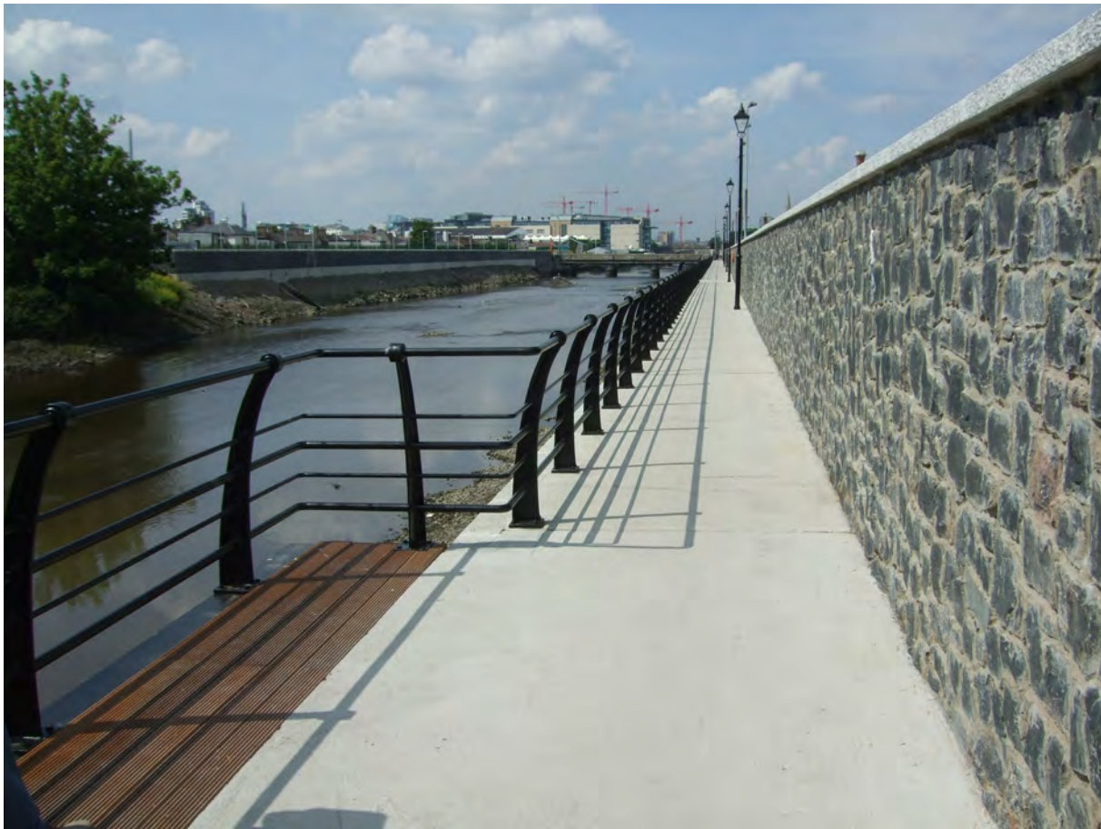
Figure 1-2: Dodder Flood Protection Scheme (Courtesy of Dublin City Council)
